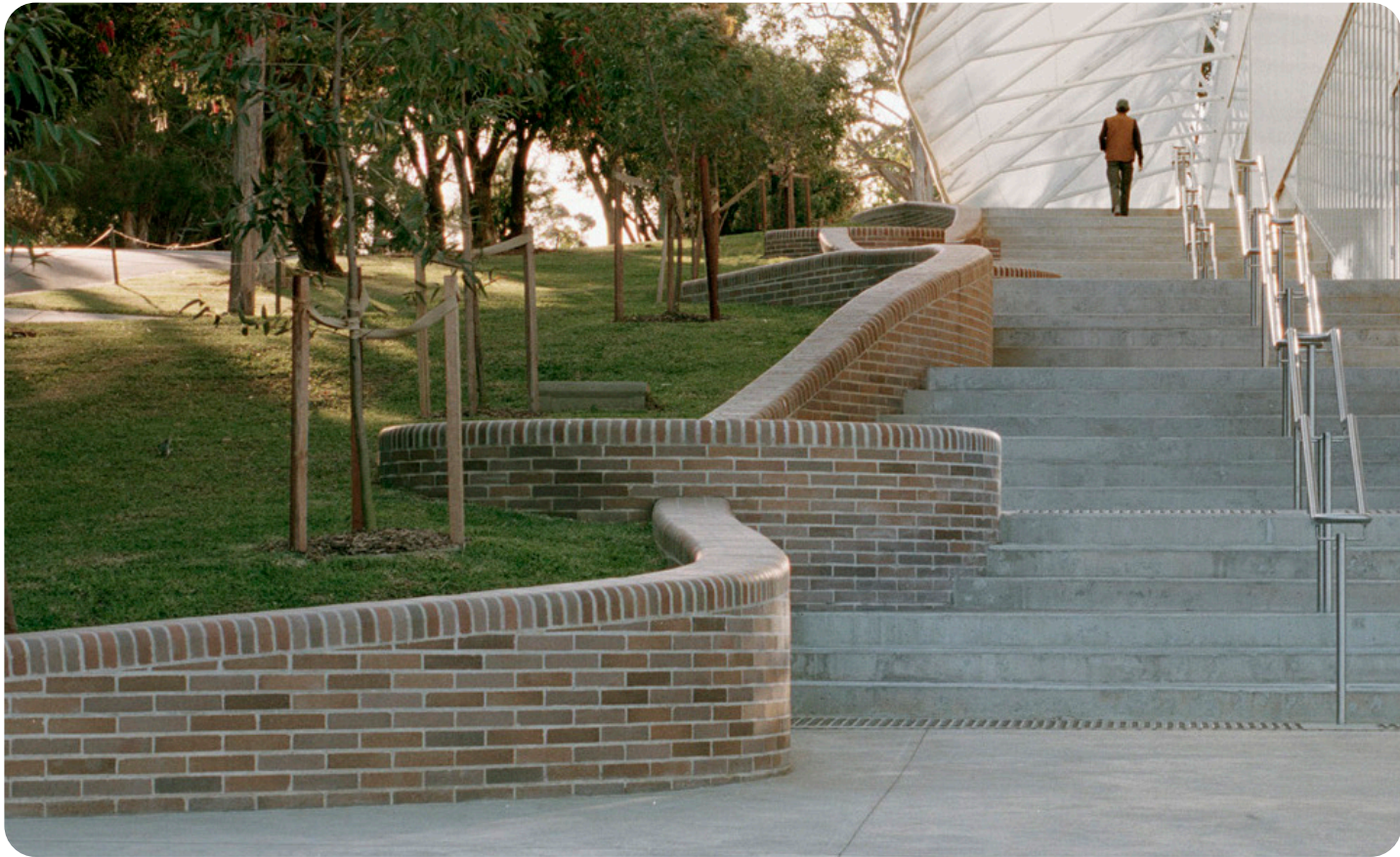
Concrete stairs with curved brick retaining walls, stainless steel handrails to centre
